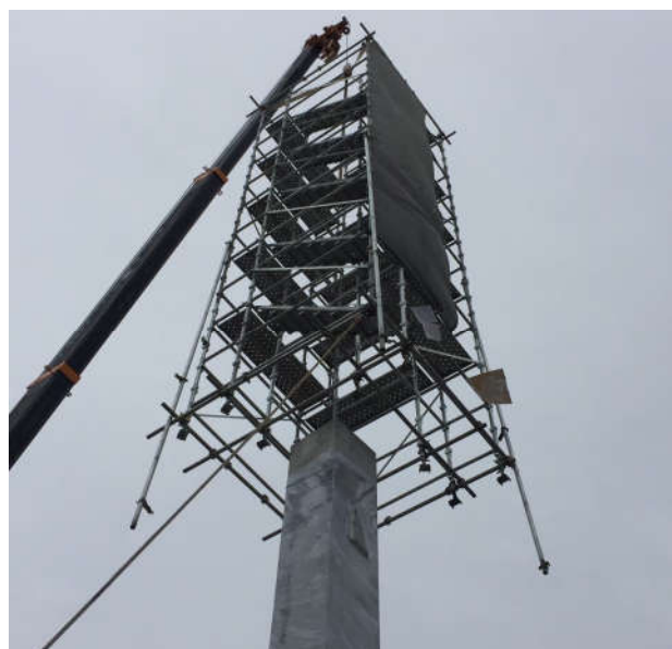
Scaffolding for column
